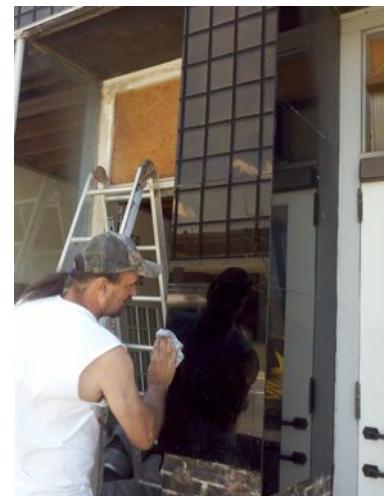
Harry Clark polishes newly installed vitrolite
